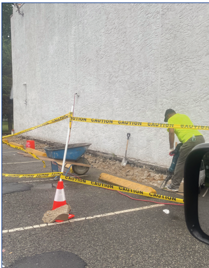
Jackhammer at work removing the old sidewalk
