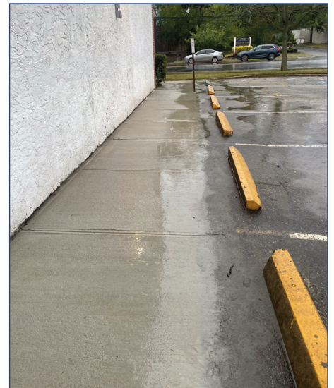
New re-graded sidewalk... note the rain graded away from building
